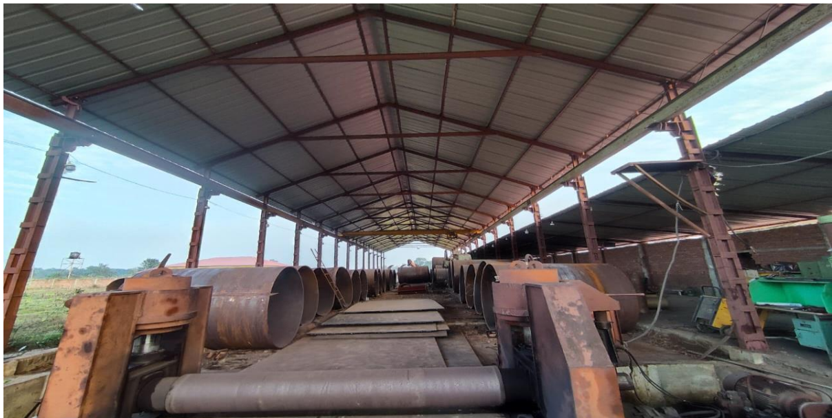
Figure: Welded pipe being stored at Butwal Workshop
