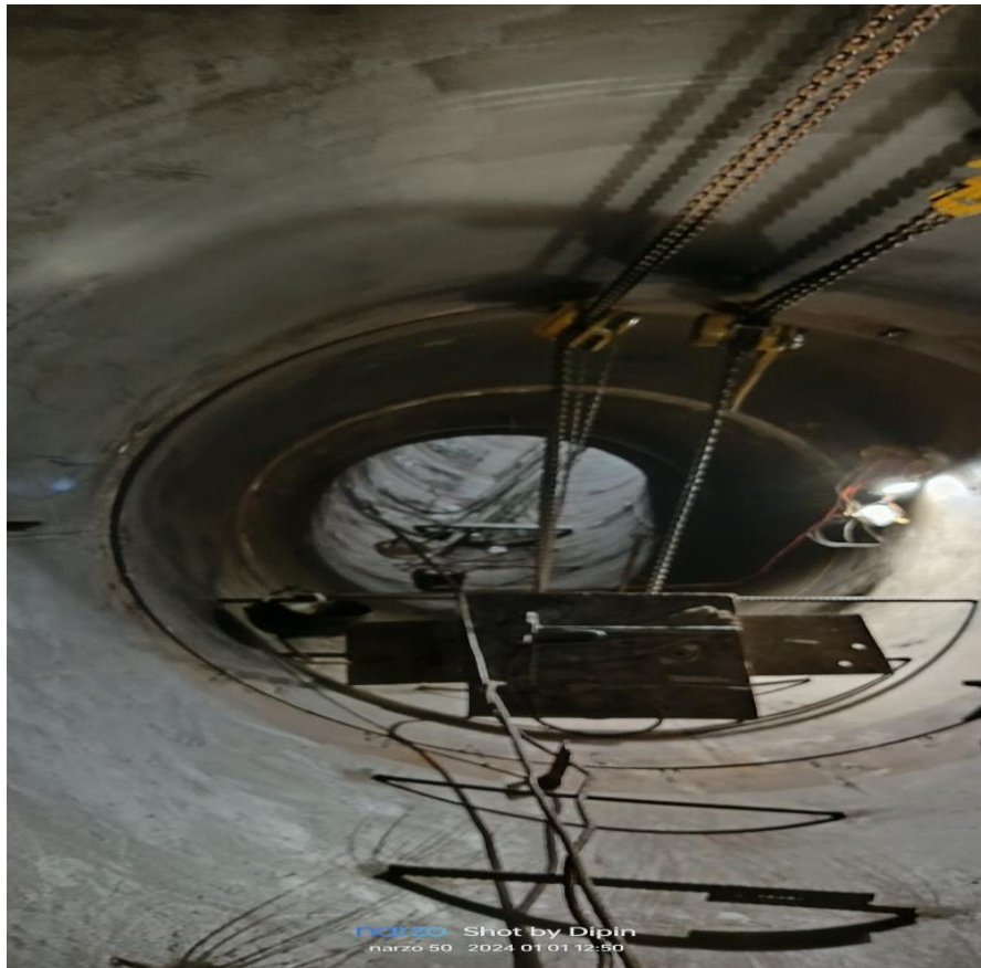
Figure: Erection of Penstock Pipes
