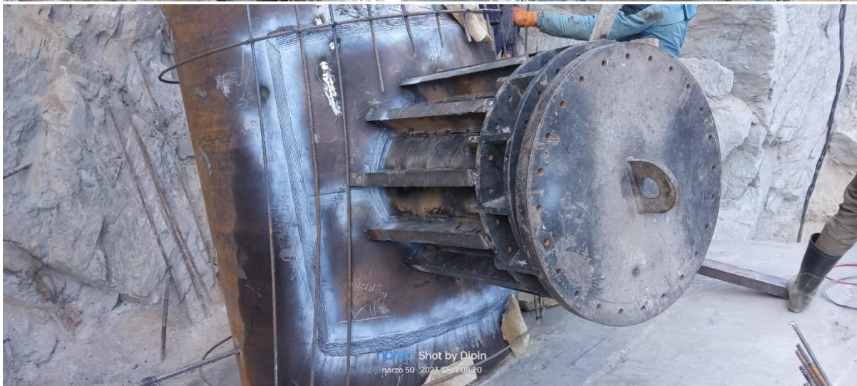
Figure: Steel Lining work and Erection of Manhole
