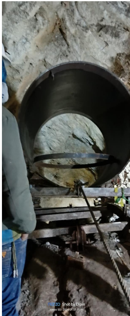
Figure: Assembly of Powerhouse Steel Partition and Lowering of Penstock Pipes with the help of Trolley
