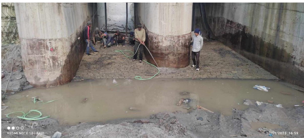
Figure: Steel lining work at undersluice area
