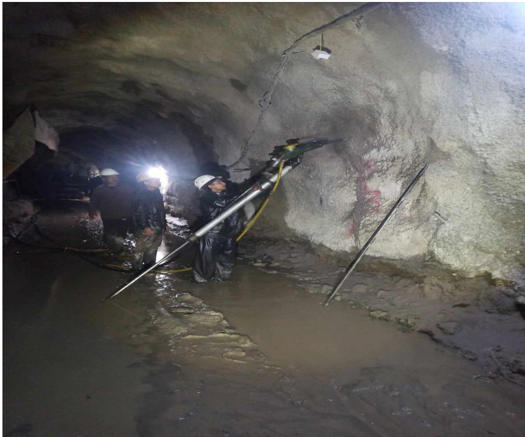
Figure: HRT hole drilling for Lugeon test
