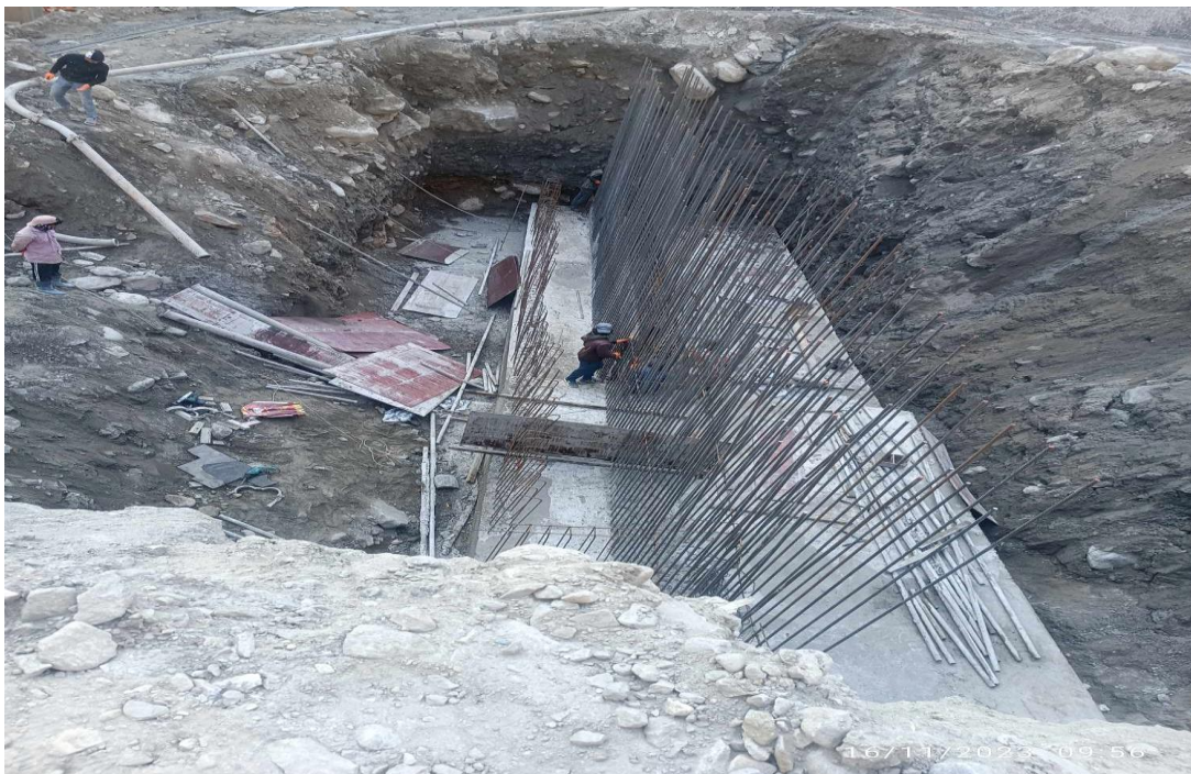
Figure: Rebar works in retaining wall of switchyard
