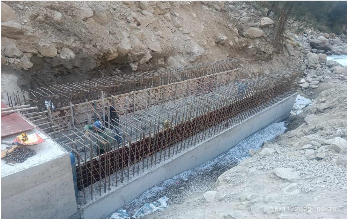
Figure: Rebar works and Formworks in tailrace outlet gate
