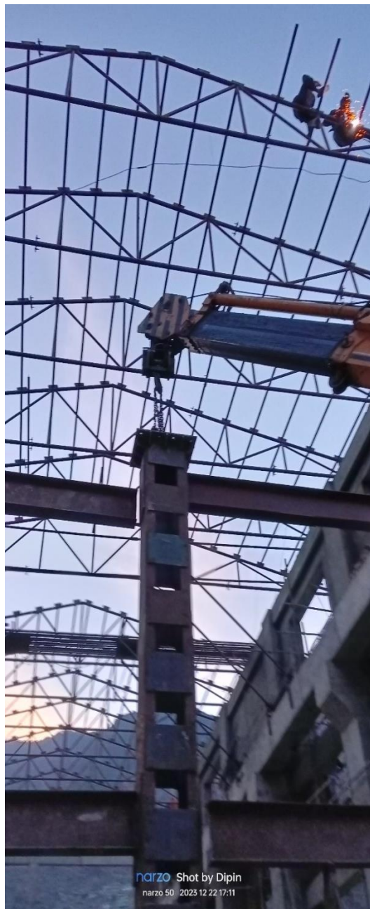
Figure: Assembly of Powerhouse Steel Partition and Lowering of Penstock Pipes with the help of Trolley
