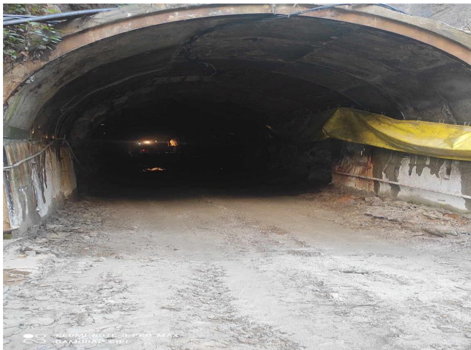
Figure: HRT invert cleaning
